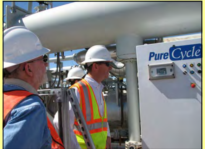
Tour and technology overview of Orrin G. Hatch Geothermal plant (credit: Utah Clean Energy)
