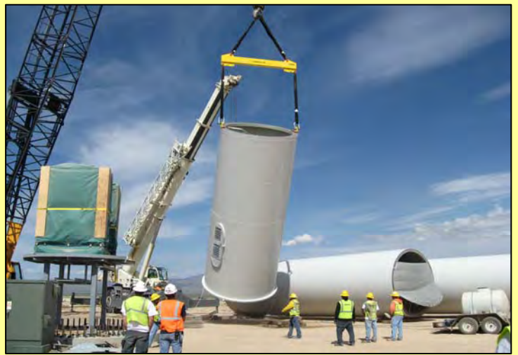
Wind turbine towers at the Milford Wind Project construction zone (credit: First Wind)
