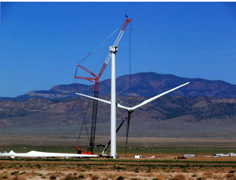
A massive wind turbine is lifted for installation at the Milford Wind Farm construction site. This wind project will be the largest renewable energy facility in Utah.
