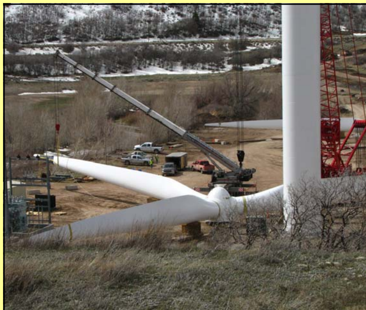
Spanish Fork construction site. (credit: Sara Baldwin, Utah Clean Energy)
