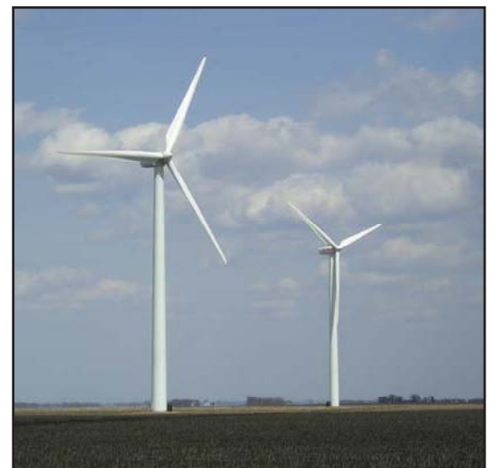
Figure 1: Three-bladed horizontal axis wind turbines.
