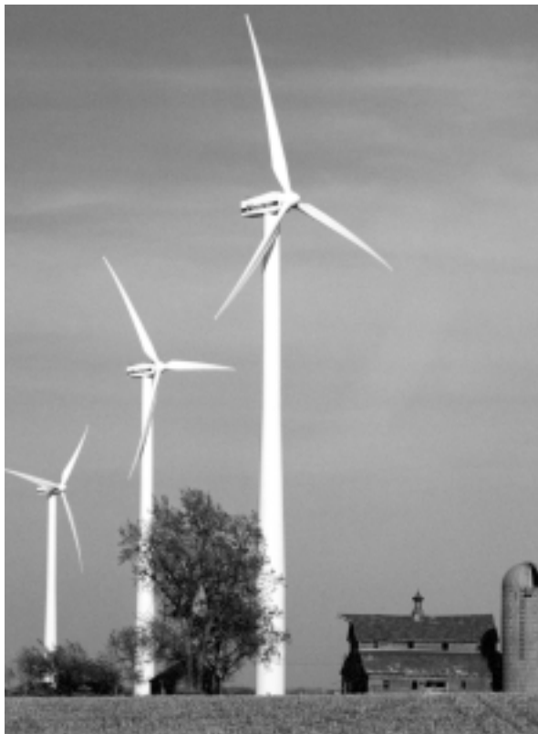
Figure 2. Today's utility-scale (900 kW) wind turbines feed clean energy to utility grids from rural areas. Photo courtesy of NREL.
