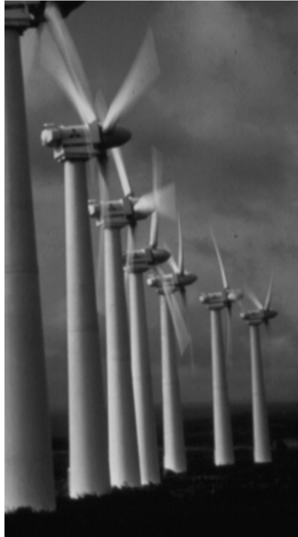
Figure 3. Tubular towers in a linear array in South Point, Hawaii. Photo by Paul Gipe.
