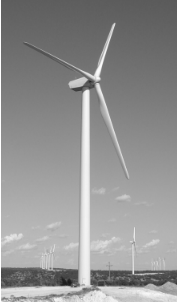
Figure 5. A large 1.5-MW wind turbine towers over a service car in Trent Mesa, Texas. The hub height for this turbine model varies from 65 to 80 meters. Photo courtesy of AWEA and American Electric Power.
