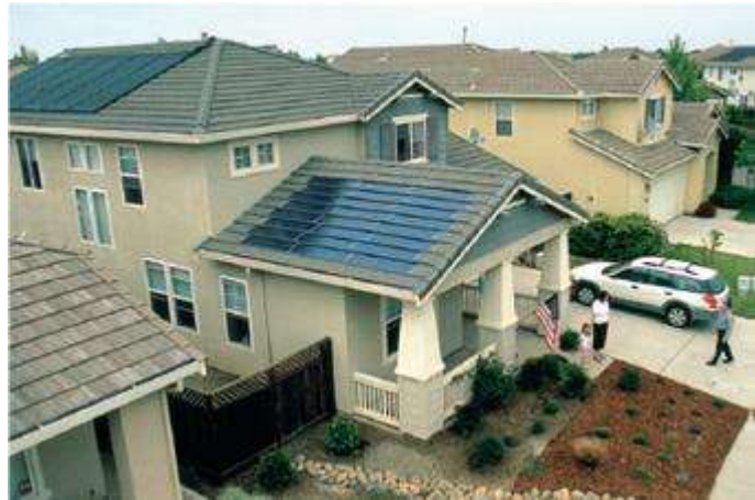
Figure 1. Example of a building-integrated rooftop solar PV system (shown on front roof) (Photo: BP Solar)
