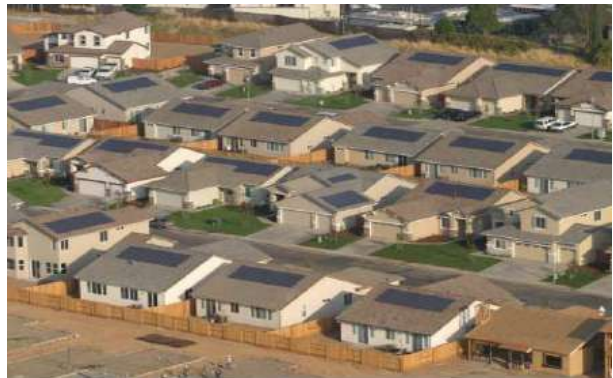
Figure ES-1. Photo of zero energy homes at Premier Gardens, Sacramento, CO (Credit: SMUD)
