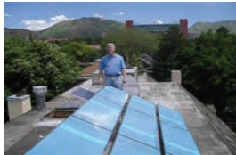
Solar Hot Water System, Utah (photo credit: Evirotherm)
